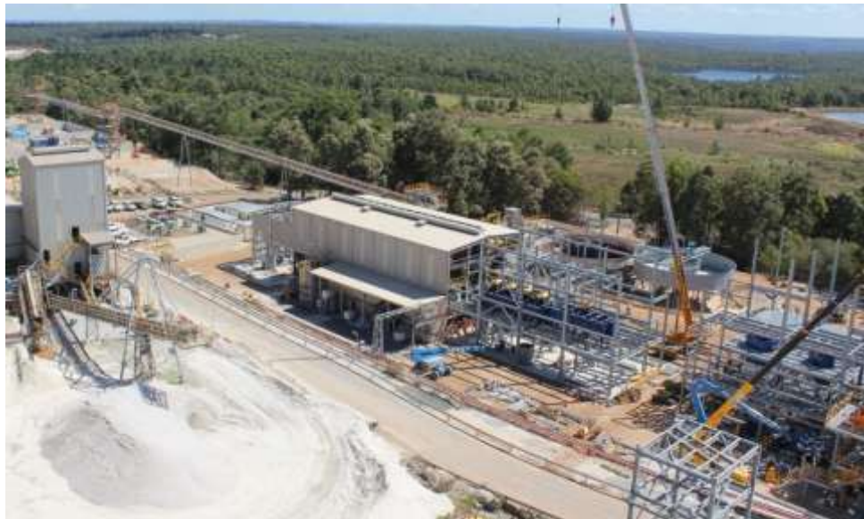
Stage 2 Expansion progress at the Greenbushes Lithium Operations
