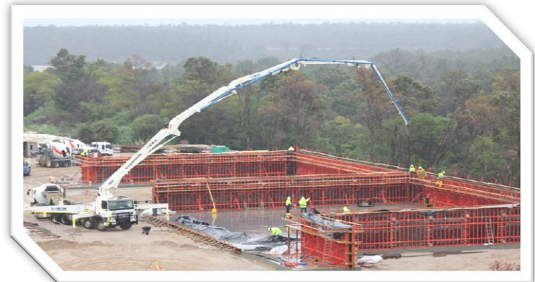
Pouring concrete for the new finished product stockpile
