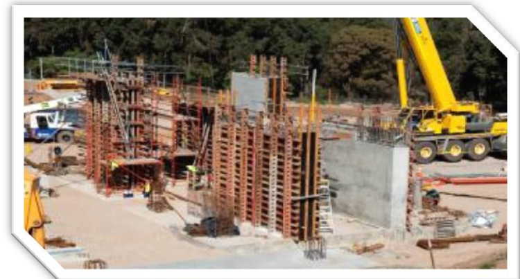
Pouring concrete for the new chemical-grade plant
